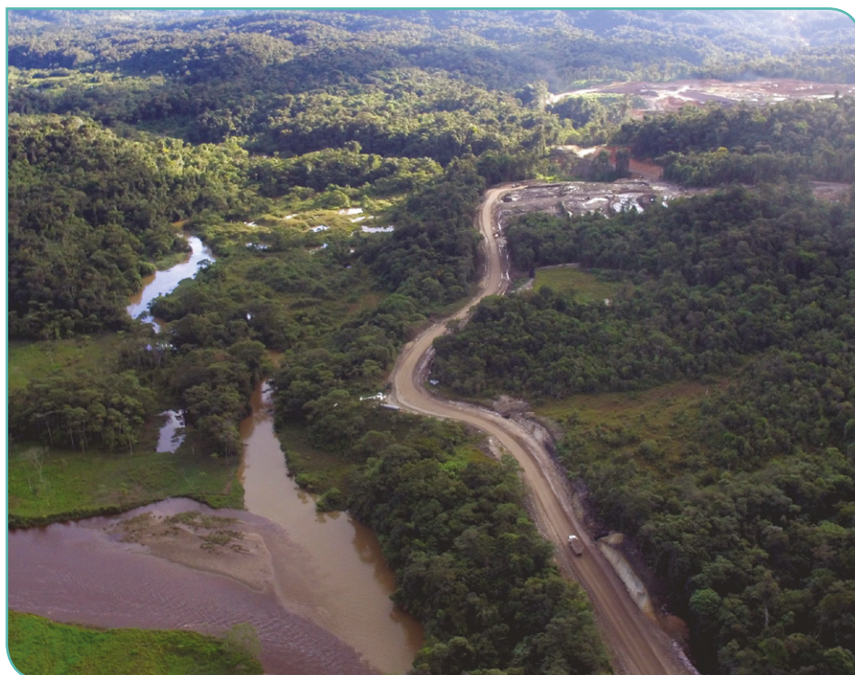
Aerial view of the North Access Road (NAR)
