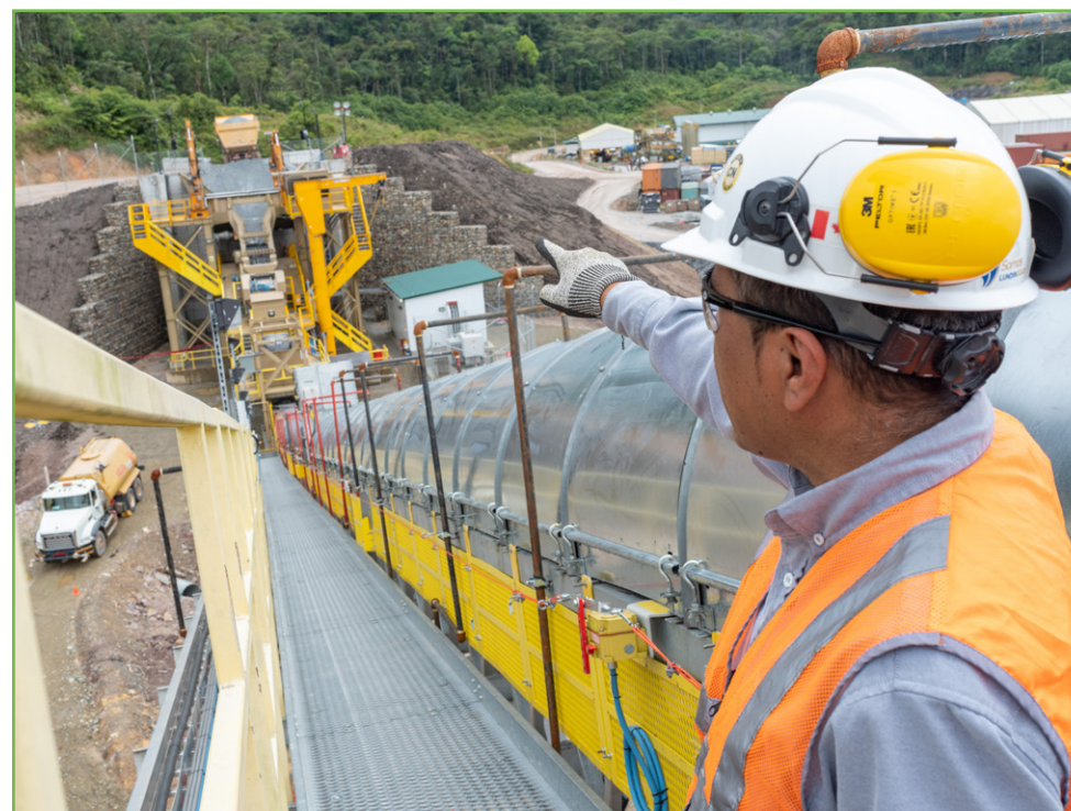
Primary Crusher, Process Plant.
